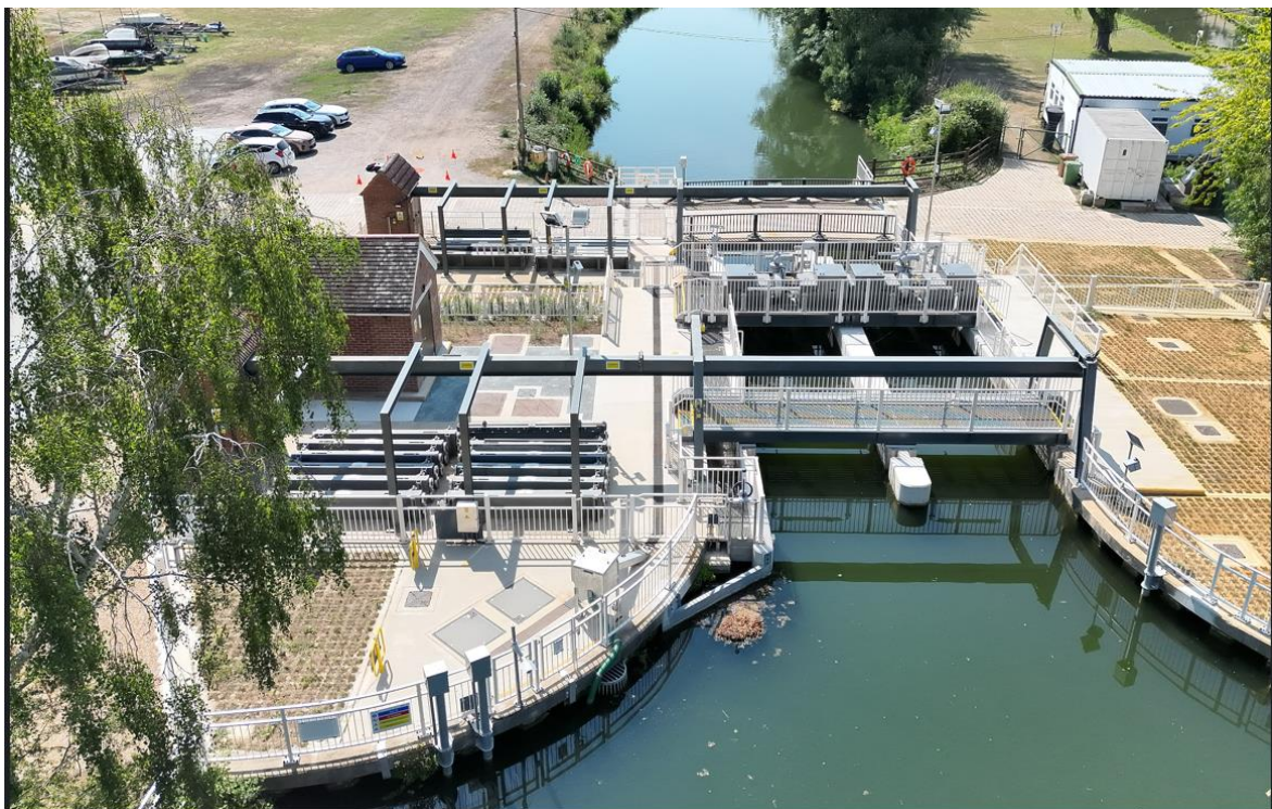
An overview of the finished works
