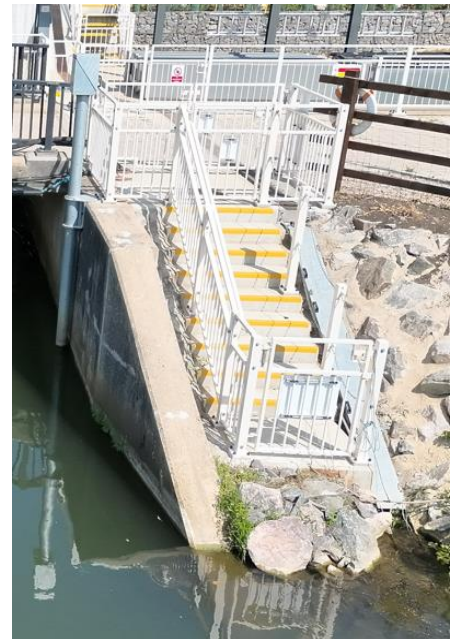
The entrance to the eel pass beside its maintenance access steps.
