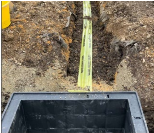
New cable ducts
