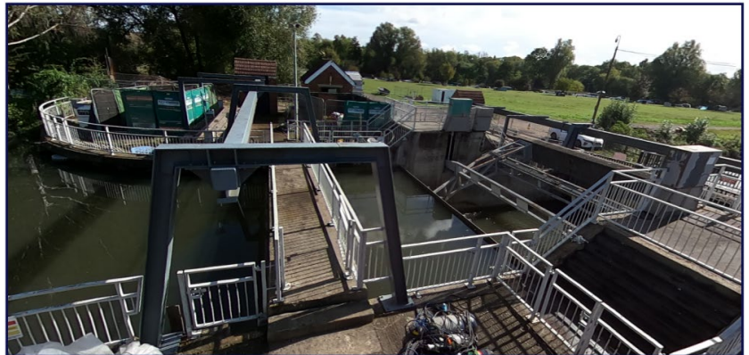
Stanstead Sluice before works started
