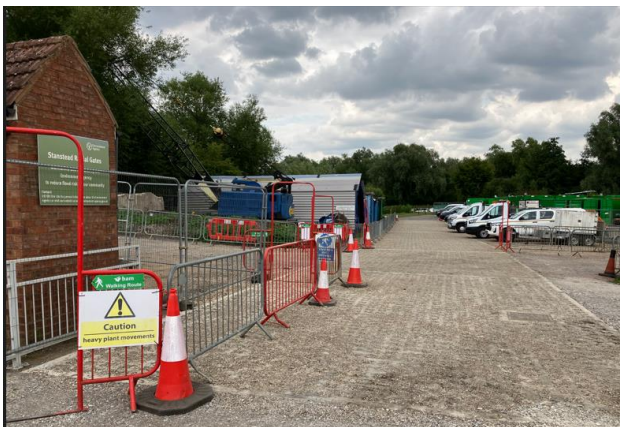
The improved tracks around Stanstead Sluice and the construction compound.
