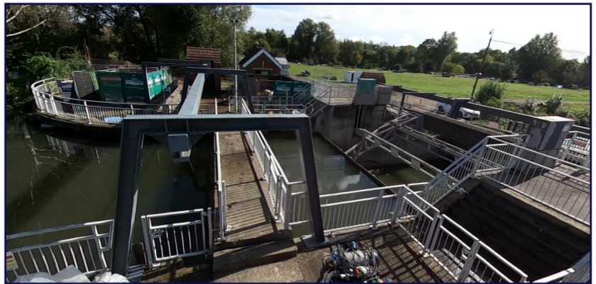
The current Stanstead Sluice
