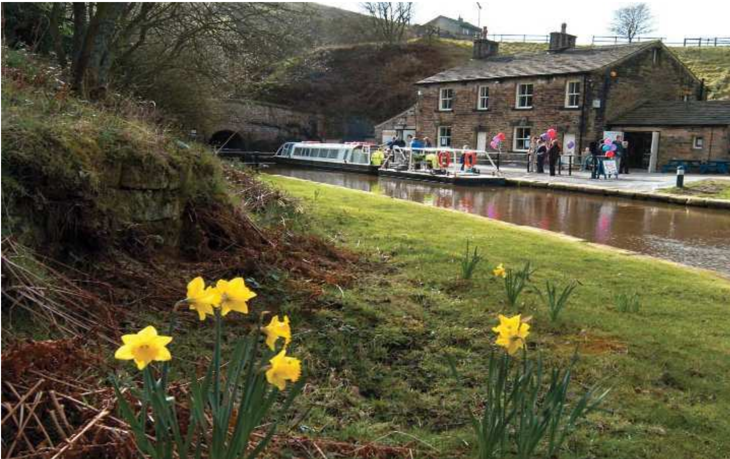
Standedge Tunnel, Huddersfield Narrow Canal
